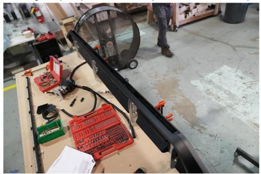
3. Slide the mRUNNER router jig over the running board making sure it is centered on the groove where the plastic trim was removed from.
